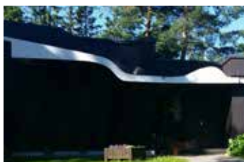
Canopy above the main entrance
